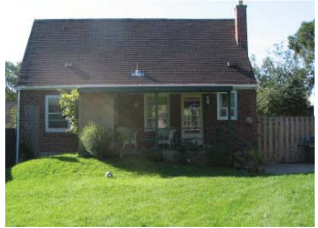
Pre-renovation: few small windows, minimal natural light.
